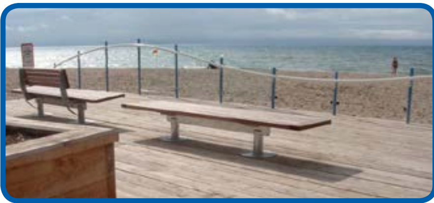
The boardwalk at Grand Bend Beach includes seating suitable for people using mobility aids and edge protection (Plexiglas within the railing design)
