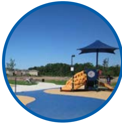
Milton Community Park: poured-in-place rubber surfacing and equipment in junior playground (photo courtesy Town of Milton)
