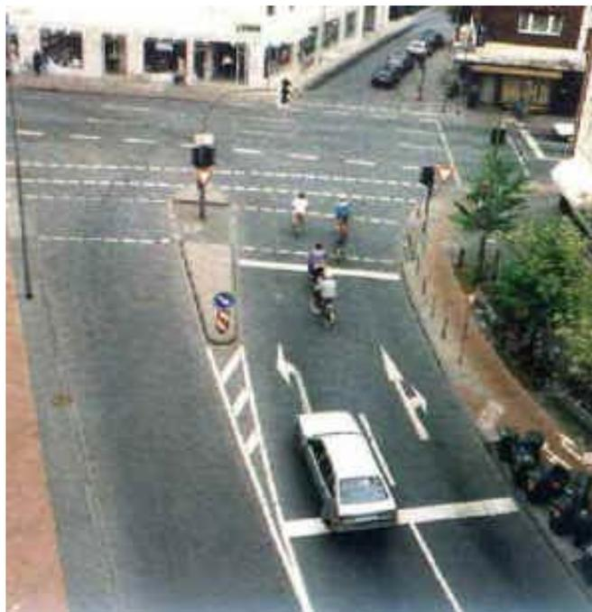
The best solution for bicycle paths is to provide separate routing or signalling that guides riders safely through the intersection.
